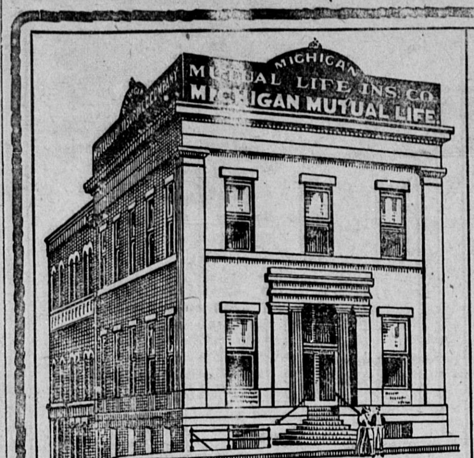
MICHIGAN MUTUAL LIFE BUILDING Corner Jefferson Avenue and Griswold Street, DETROIT
