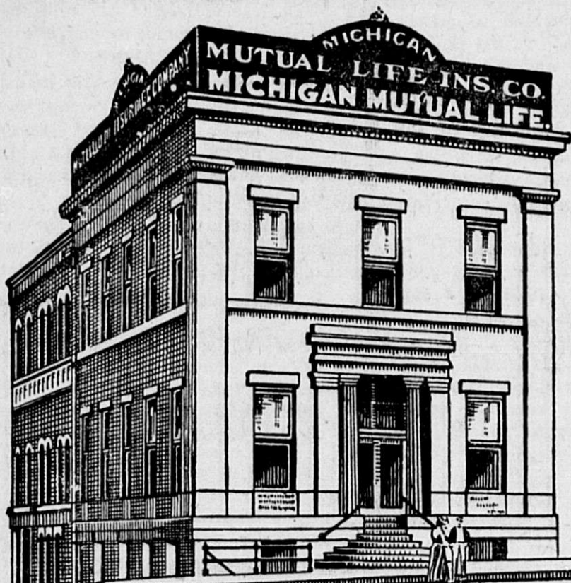
MICHIGAN MUTUAL LIFE BUILDING Corner Jefferson Avenue and Griswold Street, DETROIT
