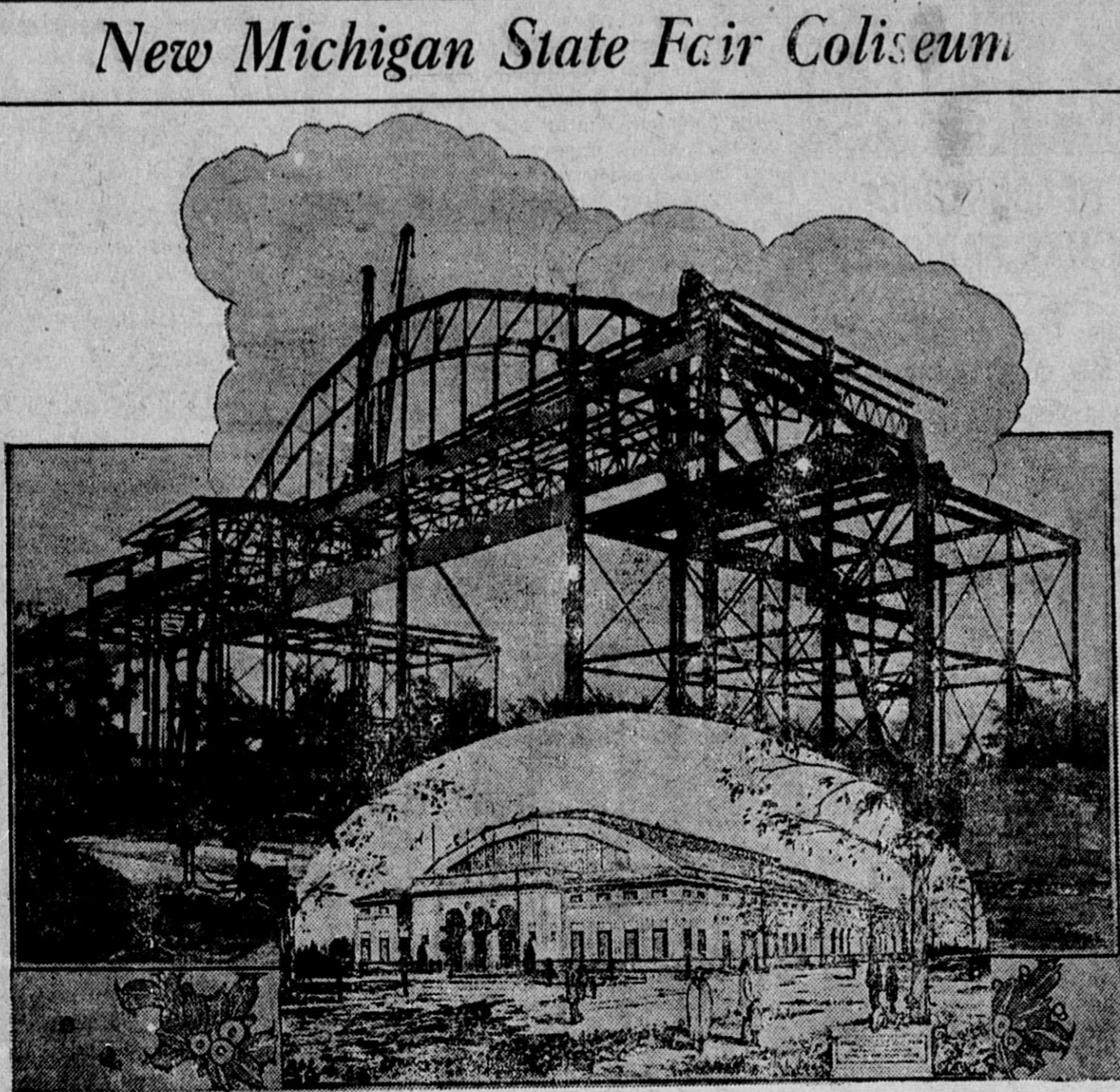
In this new $300,000 building, now under construction on the Michigan State Fair grounds at the northern outskirts of Detroit, the horse show and historical pageant at the exposition, September 1 to 10, will be staged. The building is of reinforced concrete and steel construction and is rapidly nearing completion as this picture indicates.
