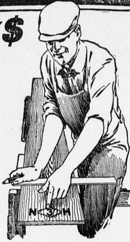
Look for the Grade-mark on end of every board or piece. Three suitable grades for structural use.
