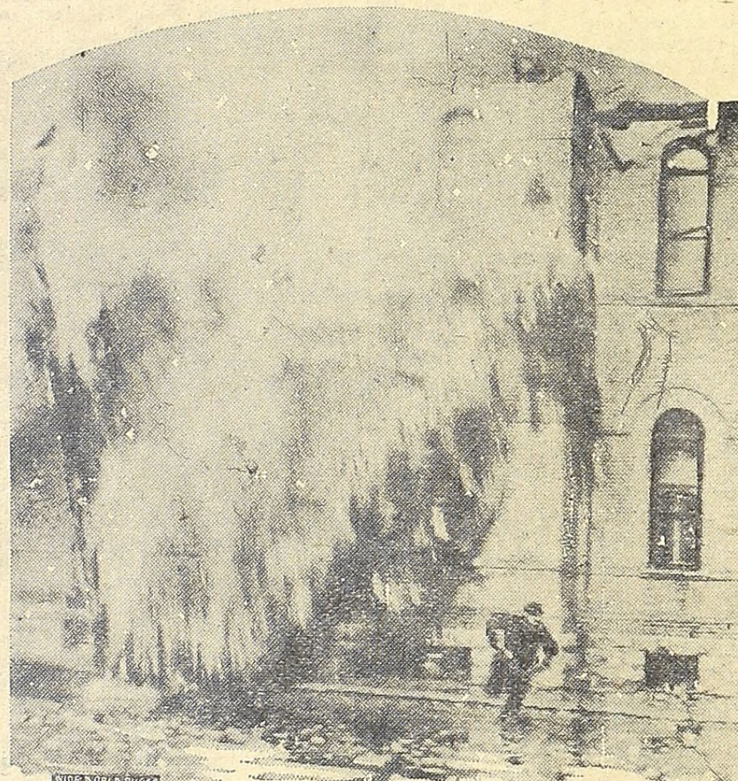
A remarkable action picture showing Fire Chief Boulden of Winnipeg, Canada, racing to escape the falling bricks of a collapsed tower on a burning Winnipeg school. The chief did not see the bricks coming, but felt a draft from above and beat it for safety.
