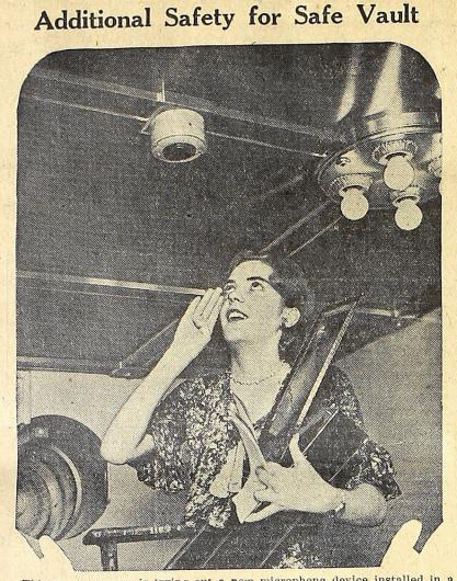
This young woman is trying out a new microphone device installed in a bank vault in Chicago. The microphone is smaller than those used in radio broadcasting and is so sensitive that a slight noise will set off the alarm, which is heard at all police stations.
