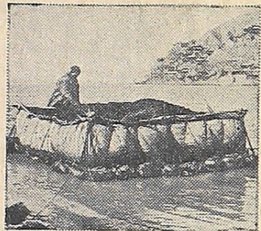
Air-Filled Sheepskins Keep This Hwang Ho Raft Afloat.
