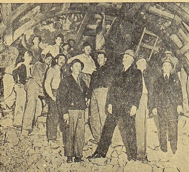
Interior of the East Coachella tunnel in California, the longest tunnel in the world, after a charge of dynamite tore out the last barrier of rock and holed-through the 242-mile-long bore. The tunnel will carry water from the Colorado river to Los Angeles.
