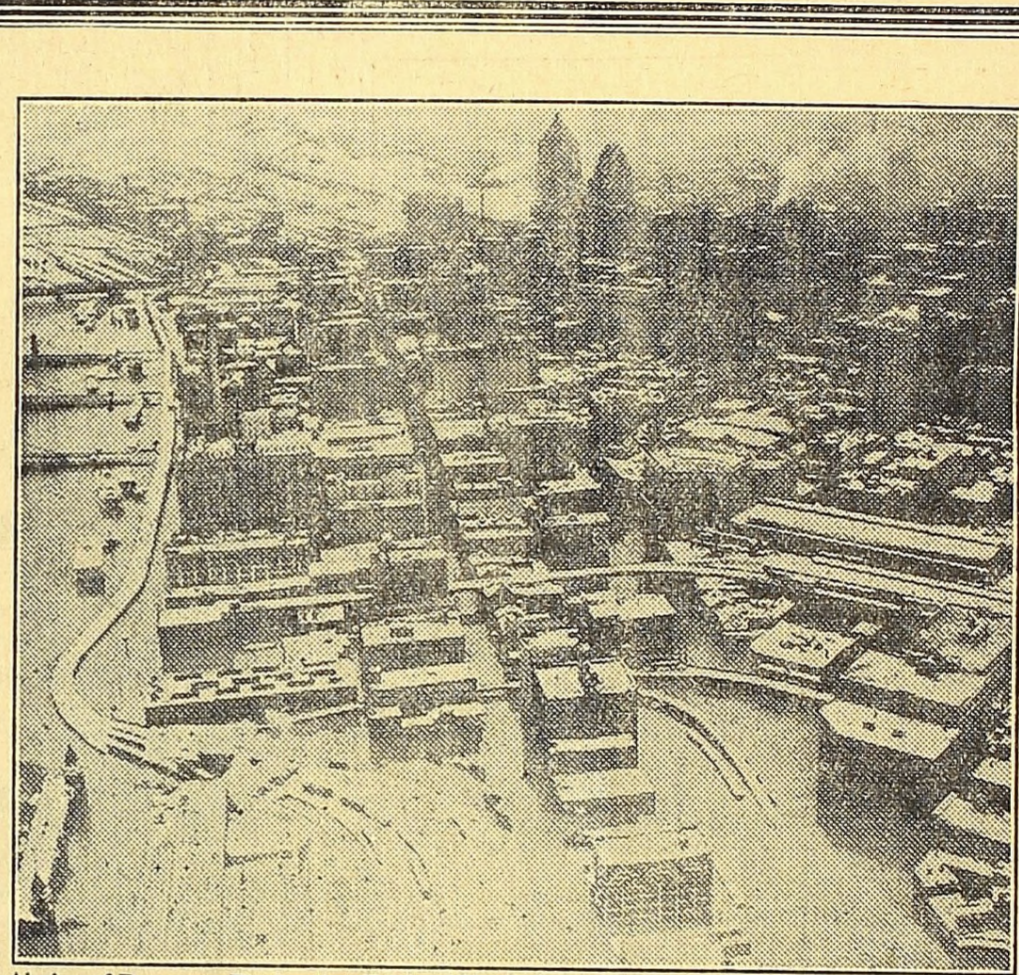
Airview of Downtown Pittsburgh at Height of Flood—International News Photo, Courtesy Detroit Times
