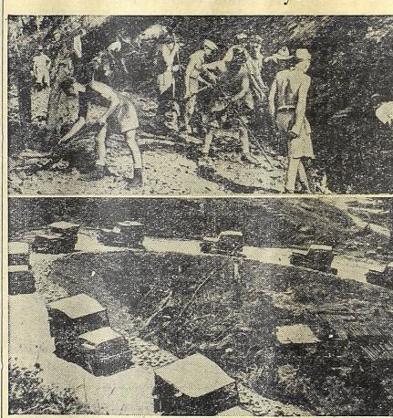
British engineers in Burma are hacking highways through jungles, mountains, to create a system of roads and supply lines over which they plan to force the Japanese from their positions in that sector. At top: British troops are working on a new stretch of road. Below: A convoy of jeeps carry supplies around a loop on a new road in Burma.
