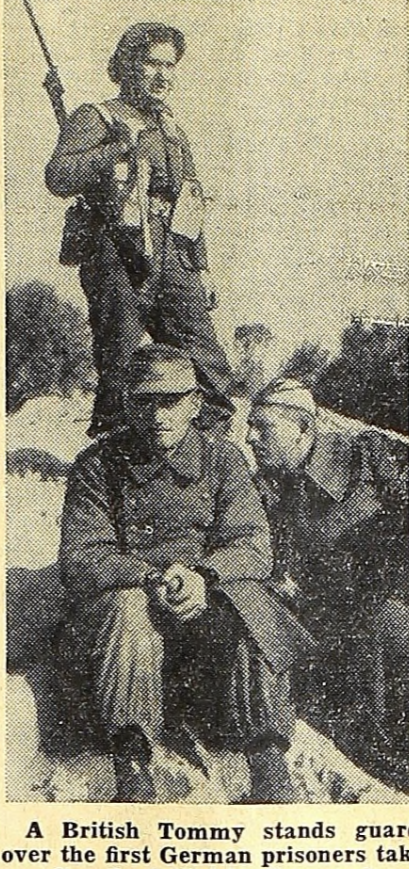
A British Tommy stands guard over the first German prisoners taken after the initial landing made on the west coast of Italy behind German lines. German forces attempted to prepare for an Allied attack on Rome by removing military equipment from that city.
