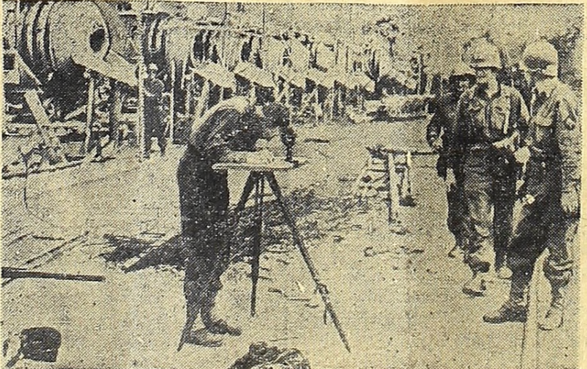
American engineers are shown surveying a 700-foot steel and concrete unfinished ramp in Normandy, which is believed to have been planned for use by the Germans as a launching site for rocket bombs. Assembly line of concrete mixers abandoned by the Nazis are in the background. Not enough and too late was the story of this Nazi effort.
