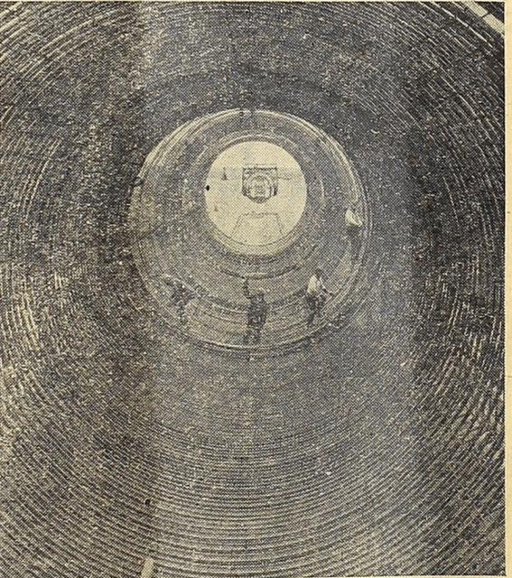
**COLUMBIA BASIN SIPHON...** Near Adrian, Wash., steel workers weave web of heavy reinforcing bars around which will be poured concrete for Crab creek inverted siphons which will convey Columbia basin irrigation water across Dry Coulee to reclaim eastern Washington sagebrush land. Twenty-five feet in diameter and 4,500 feet long, it will be world's largest monolithic concrete pipeline.
