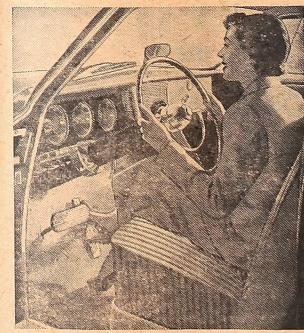
No clutch pedal, of course—and you're safe right from the start! No clutching-no declutching-with Studebaker Automatic Drive. As car moves forward, you just feed the gas, steer and brake. Your Studebaker "shifts for itself"-makes gear changes automatically, quietly and smoothly. You keep the pointer on the steering post in "drive" position most of the time. But when you switch on the ignition, the engine will start only if you have first set the selector lever at "park" or "neutral."
