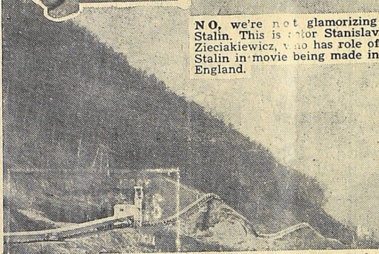
ROLLER COAL-STER , snaking over West Virginia mountains near Charleston, is a 14,000-foot-long conveyor belt designed and built by B. F. Goodrich company to haul coal to barges on Kanawha river for use in large power plant. The belt eliminates a 14-mile truck haul over mountains.
