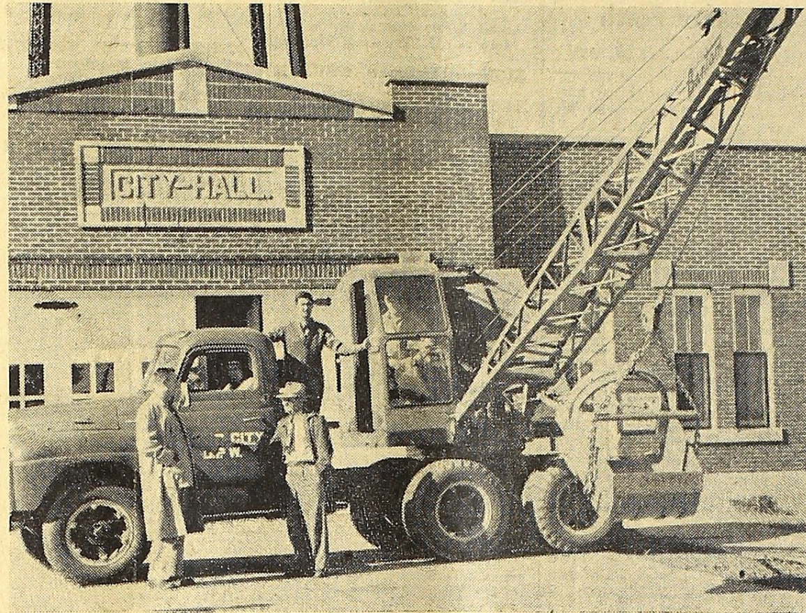
Tawas City's new dragline delivered Friday by Gordon Everett of the Ottawa Equipment Co. of Tawas City.
