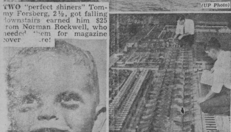
MINIATURE of plane plant final assembly area enables Republic Aviation Corp. to keep close tabs on F-84F Thunderbolt production at Farmingdale, L.I. It also aids in constant improvement in flow of materials and sub-assemblies to final production line.
