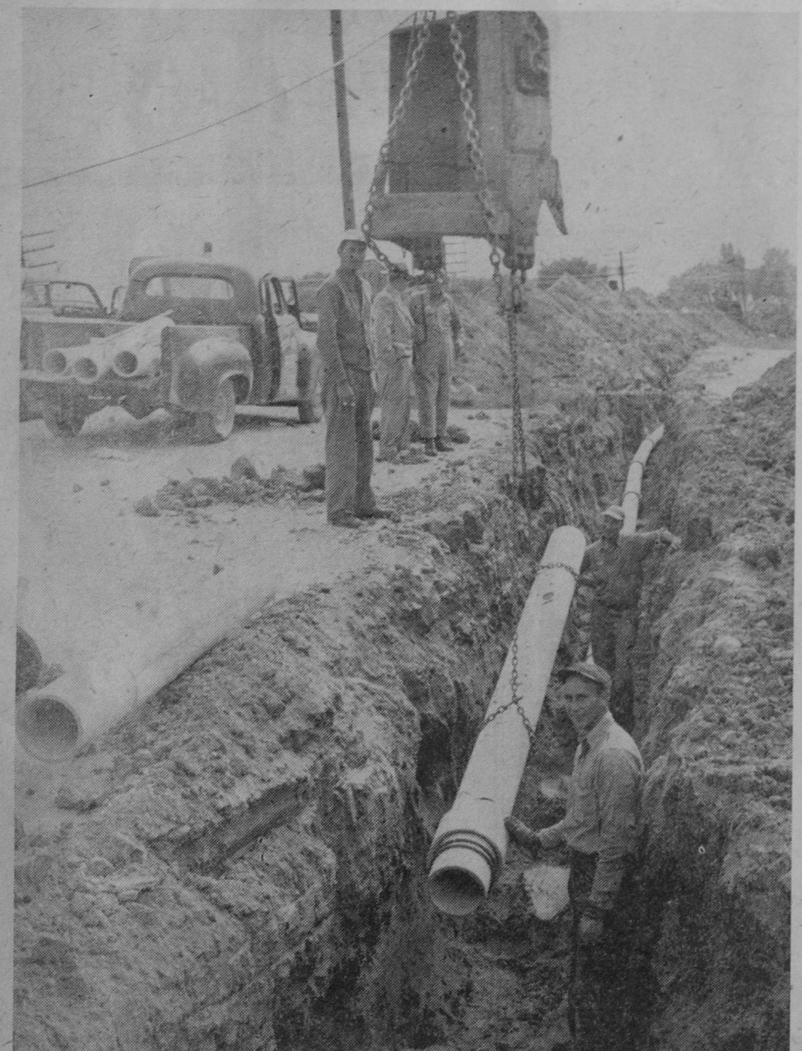
LAYING LAST SECTION OF THIRD WARD FORCE MAIN
