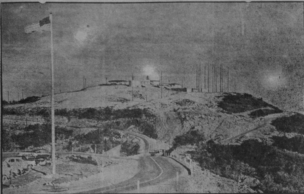
WATCHDOG MOUNTAIN — An "around-the-clock" sky watch is kept to guard the San Francisco Bay area from surprise air attack. The $5 million U. S. Air Force radar center on Mount Tamalpais picks up unidentified planes on radar screens and relays the information by radio to fighter headquarters at nearby Hamilton Field. The ball-shaped sphere at center stands 65 feet high and houses radar antennae. Wooden poles at right are 90-foot-high radio antennae towers.
