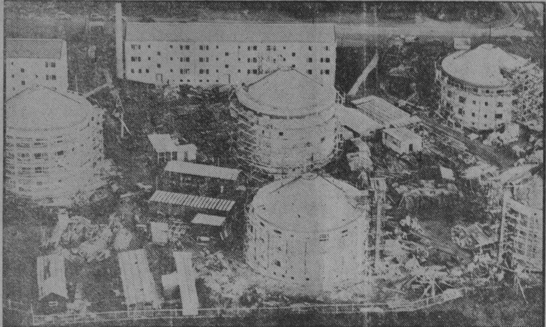
'ROUND THE FAMILY CIRCLE—These unique circular apartment houses are under construction in a Stockholm, Sweden, suburb. The new-type buildings contain 10 one-room apartments on each of their four floors, the rooms being placed fan-shaped around a large, circular staircase. Each of the houses will be painted a different color.
