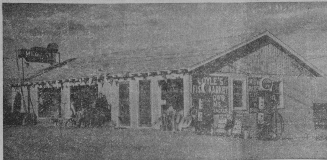
The new home of Mid-West Hardware and Supply and Coyle's Fish Market in Tawas City. This new building, owned by John Coyle of this city, was recently constructed on US-23. Coyle is the new distributor for Speedway Petroleum Products in this area—Herald Photo.
