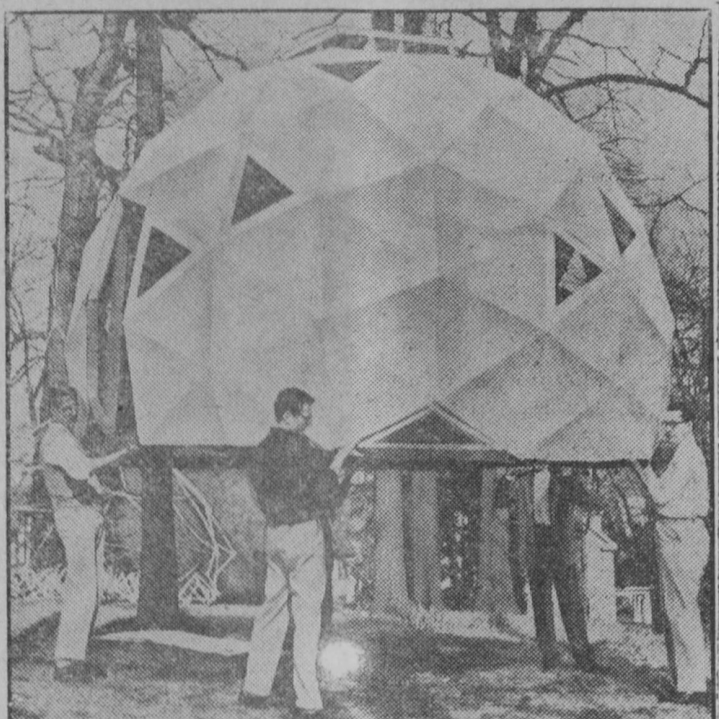
CARDBOARD VS. H-BOMB—So light that four persons can handle it, this experimental cardboard air-raid shelter is set in place on the campus at Ann Arbor by students of the University of Michigan. The collapsible, domed shelter could be mass-produced. Designer Richard Fuller believes it could better withstand H-bomb shock waves than could conventional shelters.
