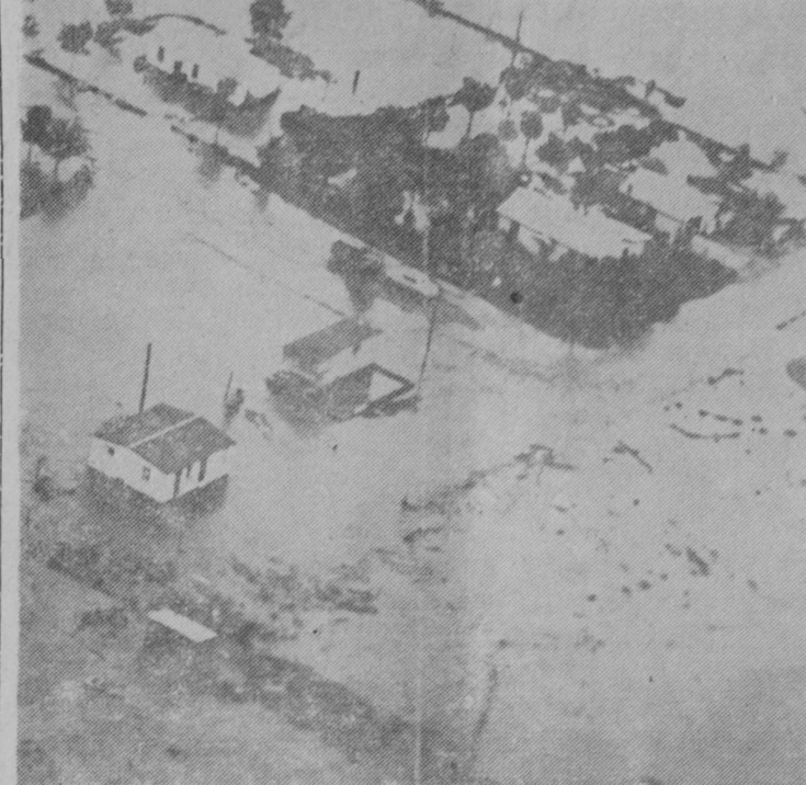
Aerial view shows water of the Pecos River as it flooded Artesia, New Mexico. Three persons have been reported drowned and eight others are still missing in the flood. Damage has been estimated in excess of one million dollars.
