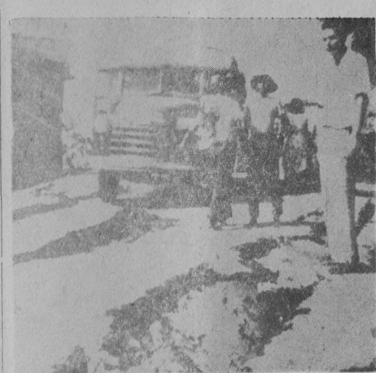
Buses halt on national highway after a series of heavy earthquakes on the island of Mindano in the Philippines, as wide cracks appear in the pavement. At least 164 deaths and millions of dollars of property damage have been caused.
