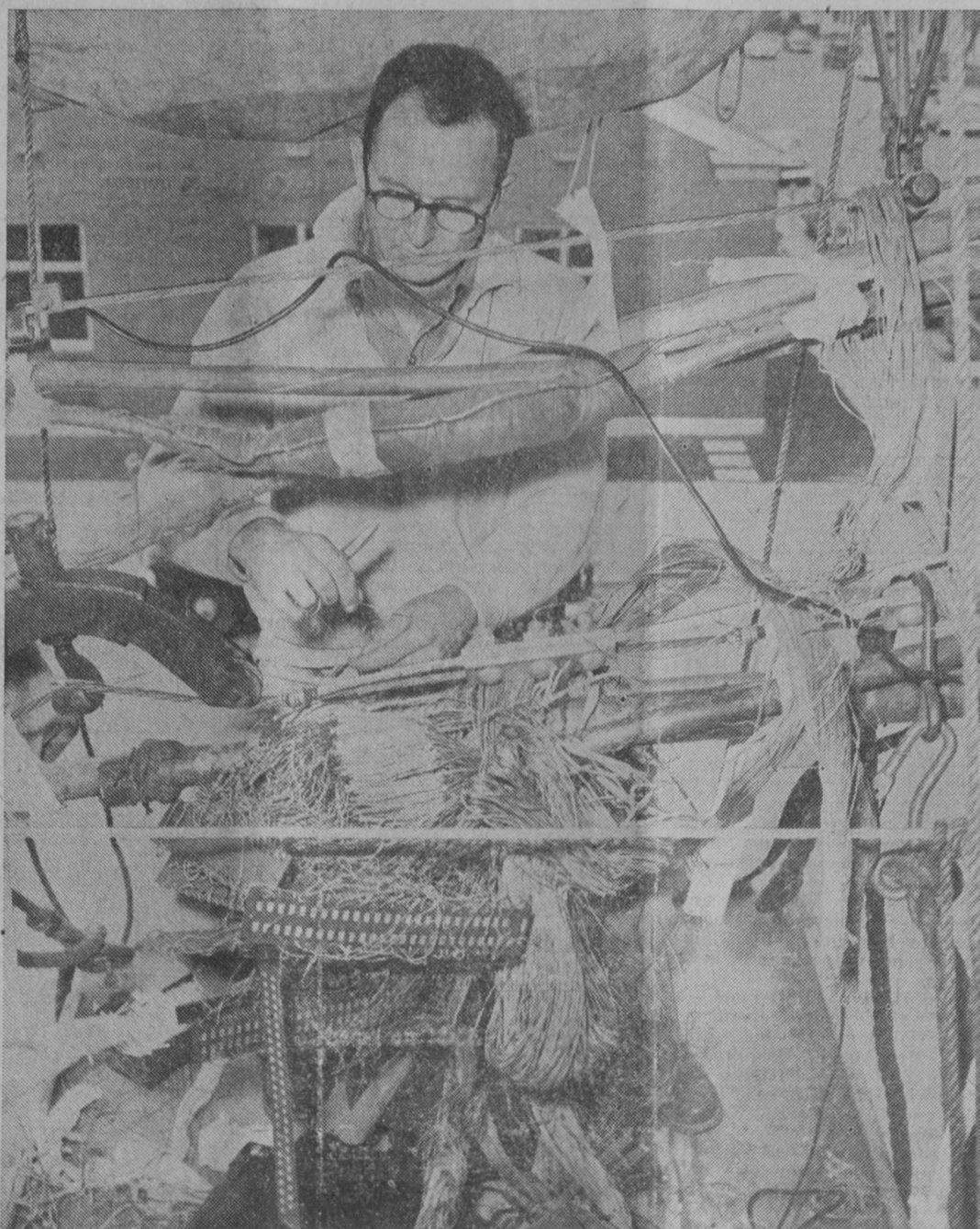
The vital and painstaking job of splicing hundreds of connections in the main cable from the new dial telephone office to serve Tawas City and East Tawas soon is being done by Michigan Bell Telephone Company Splicer Donald G. Fox of Bay City, Michigan. Bell cutover crews have been in the Tawas area for months preparing for the introduction of dial service here June 19.
