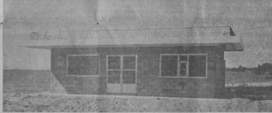
Shown above is the new Tawas City Park Concession building owned by William Borosh and Gordon Clute of this city. The 30 by 16 foot building is of cement block construction. It will serve as a ticket office for the charter boat at the dock, bait shop and hamburger drive-in.
