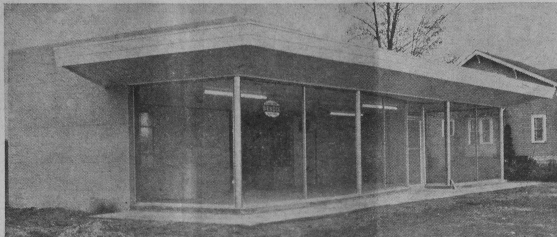
Pictured above is the new 50 by 25 foot salesroom of Fuelgas Company, Incorporated, in Tawas City. Constructed of concrete and steel, the building has a solid plate glass window front. Grand opening for the new building will be held next week.—Tawas Herald Photo.
