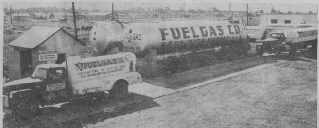
DEPENDABLE SUPPLY —Our huge 30,000 gallon tank, which holds enough LP-Gas to heat a five room house for 20 years, assures you of a dependable supply.
