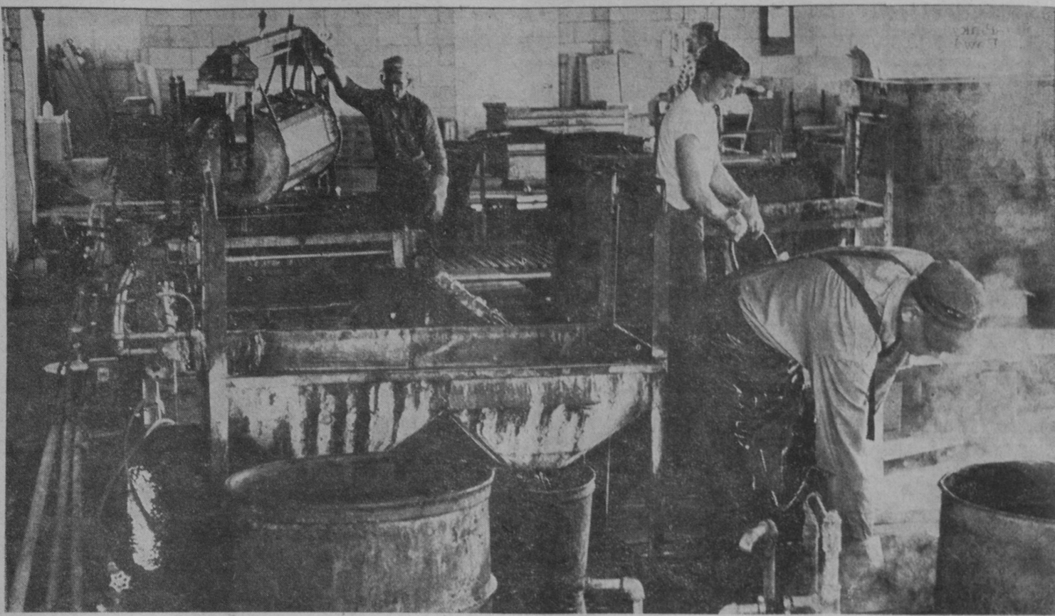
Pictured above is a view of the interior of the new Tawas Plating Company plant in Tawas City showing workmen transferring metal parts to the different solutions in the electroplating process. The workman at the left is operating an overhead hoist which moves plastic barrels containing parts to the deep tanks. Steam rises from the final cleaning bath at right.—Herald Photo.
