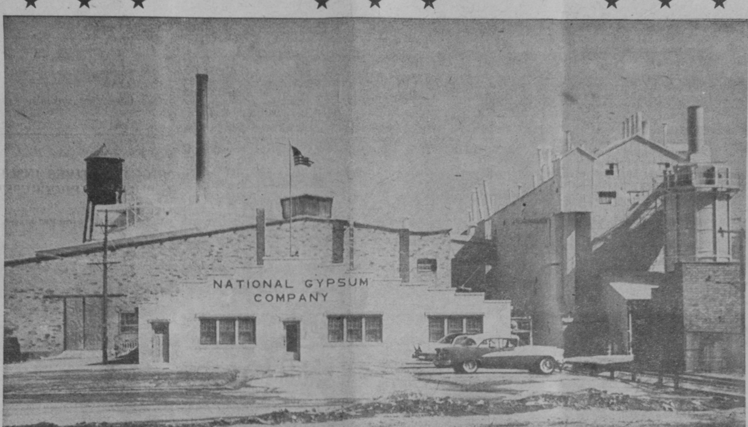
The National Gypsum Company announced last week that the Tawas area and Isoco County would take part in the company's $90,000,000 expansion program. Pictured above is a view of the National Gypsum plant in Sherman Township which employs 350 men. Constructed 27 years ago, the plant produces gypsum board and other gypsum products for shipment to the midwestern area by rail and truck.—Tawas Herald Photo.
