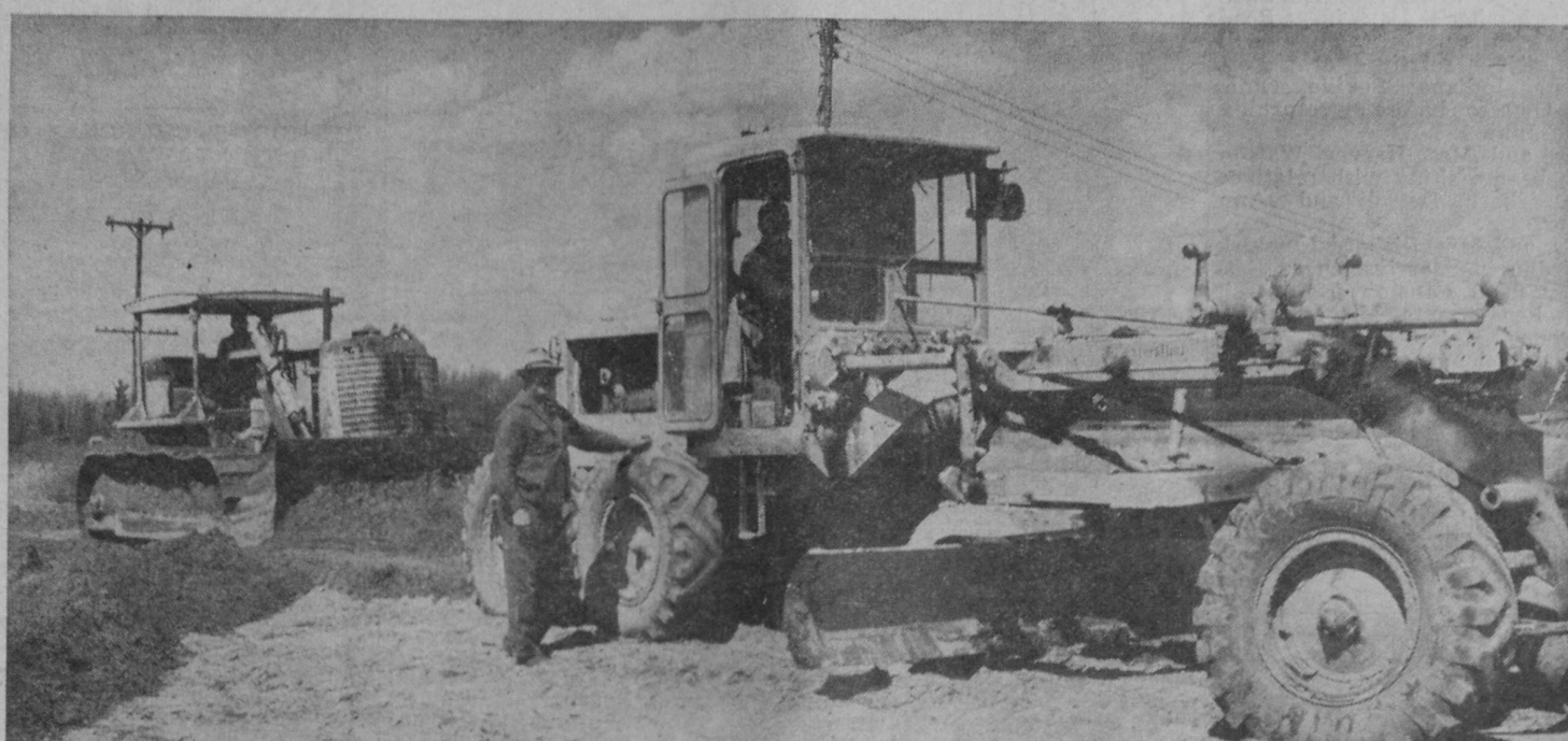
WORK STARTED LAST SATURDAY on rebuilding the Wilber Road from the corner of M-55 to Miners Corner on the Monument Road. In the above photo, Rudy Anderson, general foreman of the Iosco County Road Commission, checks progress on the job with Elmer Bischoff, grader operator, and Harold Funk, shown operating the bulldozer. Mr. Anderson said that about 14,000 yards of fill would be required to bring the road to the proper grade. After the road is graded, it will receive a single-seal coat. Plans call for blacktopping next year. Work on the road is expected to be completed by the middle of July.—Tawas Herald Photo.
