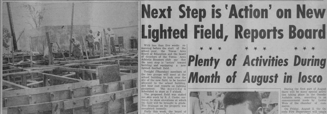
PROGRESS ON East Tawas' new water filtration plant is pictured above. Workmen are shown preparing wooden forms in which concrete will be poured for the 62 by 12-foot clear well, or water
