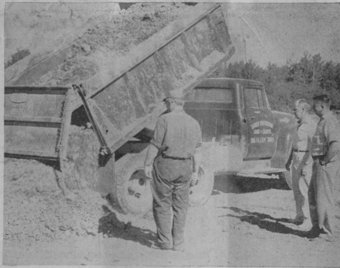
ONE OF THE FIRST truckloads of clay hauled to the new athletic field Saturday is shown above. At left is Supt. Reynold Mick, with Dr. E. B. Cavell and Cecil Cable at right.—Herald Photo.
