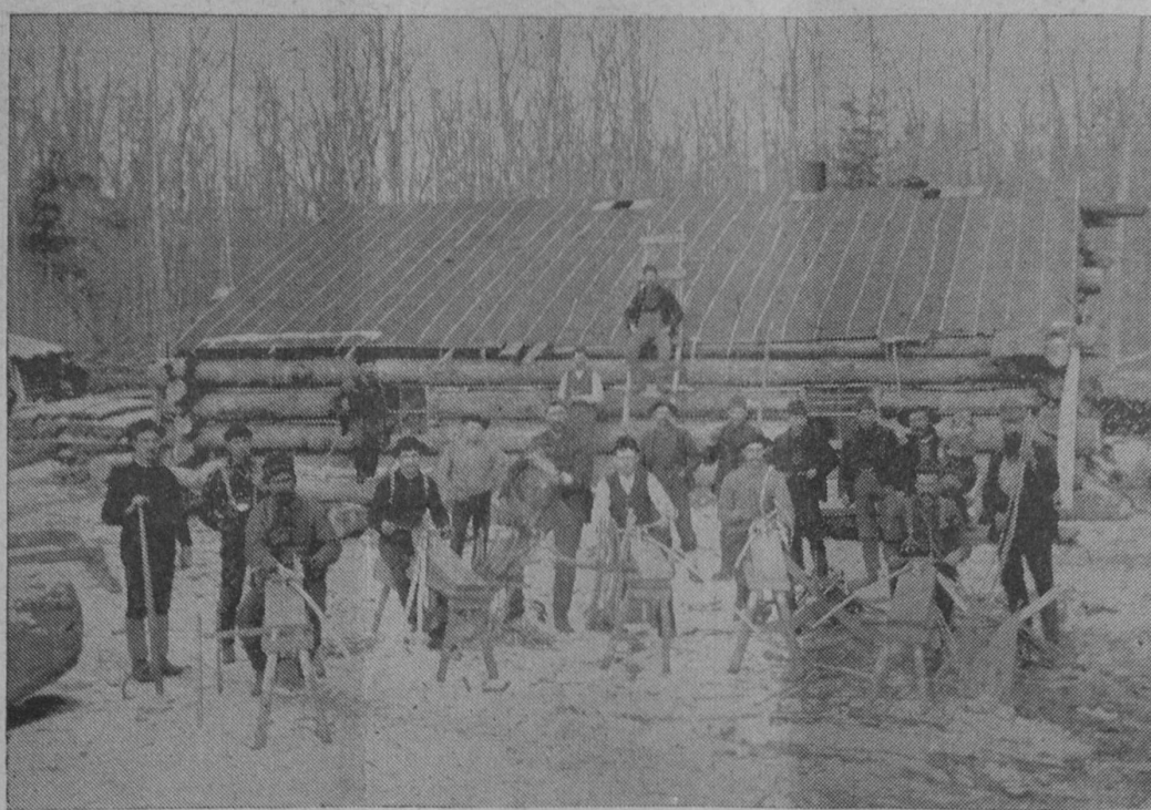
PICTURED HERE is a crew of men making barrel hoops in a hoop yard in Sherman Township about 1870. Black and white ash were used for the hoops, which were hand shaved. Matthias Schneider, who was the first supervisor of Sherman Township, was owner of the yard. The picture was furnished by his son, Anthony Schneider, who is a resident of Burleigh Township.
