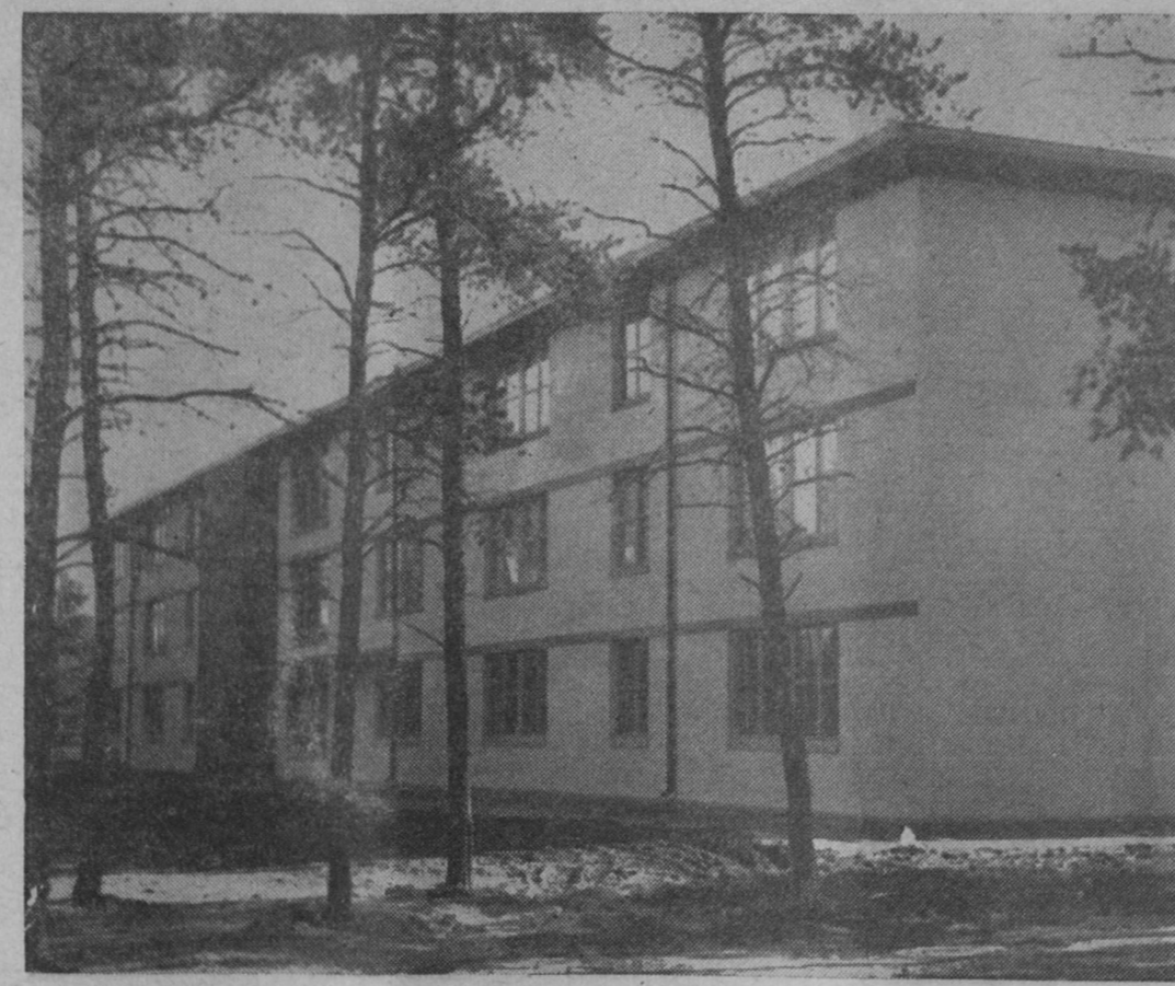
ANOTHER NEW DORMITORY for Wurtsmith airmen was ready for occupancy last week. The 200 man unit, similar to Husted Hall, will be designated building No. 520. The new dormitory was erected by Peterson and Westberg Construction, Cadillac, at a cost of $311,430. It becomes the home of airmen assigned to the 31st FIS, the Wurtsmith squadron equipped with the supersonic F-102A interceptor. Two three-man rooms are separated by a modern shower and bathroom. The dormitories are designed to provide the maximum in modern living comfort for today's airmen. Thus, the name "dormitory" is replacing the old idea of "barracks." Buildings such as Husted Hall and 520 are definitely not barracks. They contain special snack bars, TV rooms and day rooms, a far cry from barracks living of previous years.—Air Force Photo.
