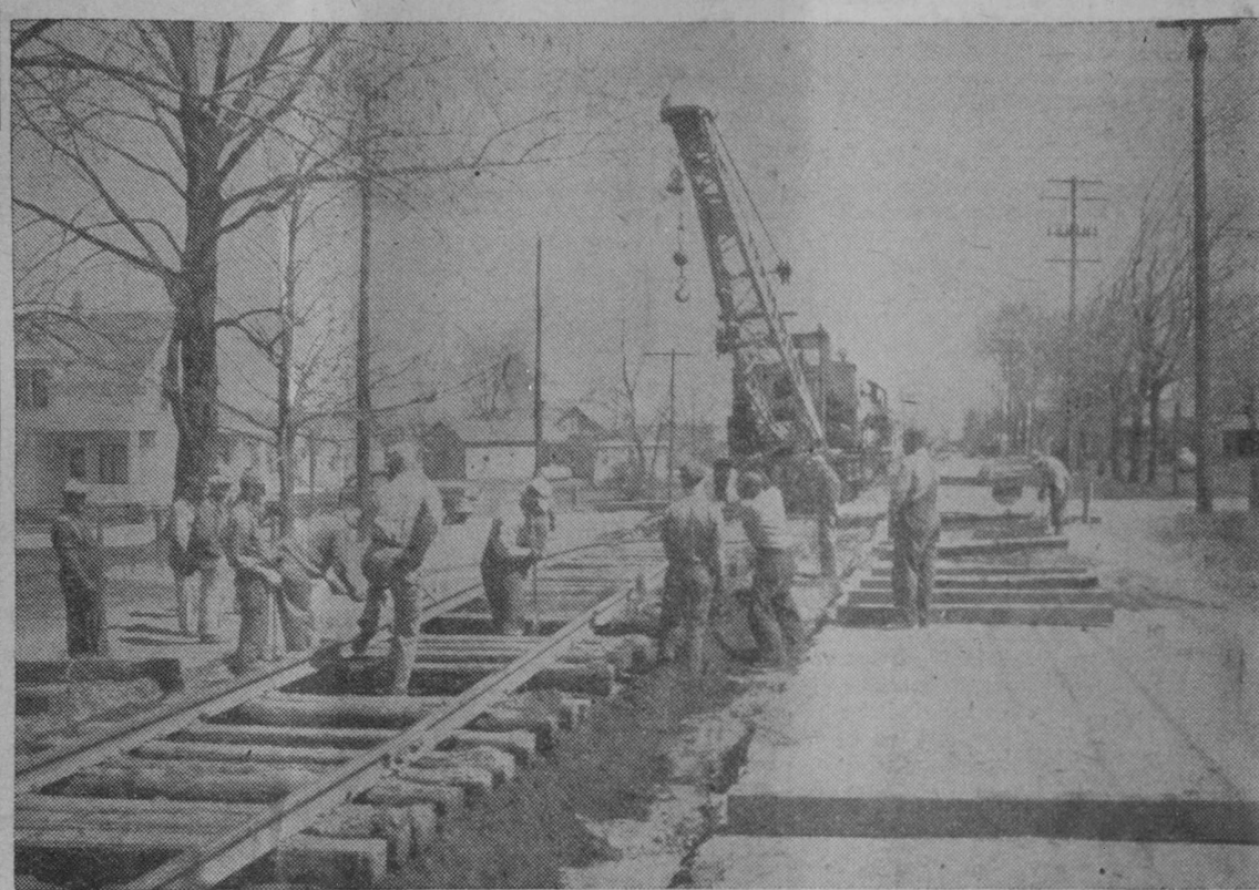
MODERN METHOD of re-ballasting tracks by the Detroit and Mackinac Railway Company is pictured above. The dragline in the background pulls an under-track plow, lifting rails and ties in one operation, at the same time removing an accumulation of dirt and old ballast. Crews following behind replace ties and respike the rails to the track. The picture was snapped as the operation moved along Court Street in Tawas City.—Tawas Herald Photo.
