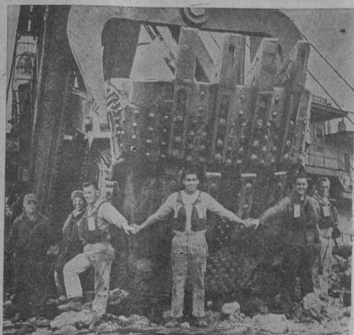
GIANT PANAMA DREDGE —This huge dredge, which was built for use in the construction of the Panama Canal, is scooping out a deeper channel in the Detroit River in preparation for the St. Lawrence Seaway. Crew members of the dredge demonstrate the size of its 22-ton bucket, which can gobble 15 cubic yards of river bottom at a bite.
