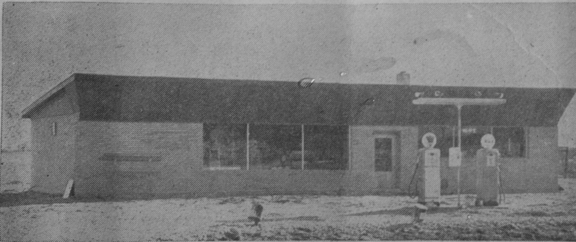
PICTURED HERE is the new Herriman Store on M-55 near the Sand Lake Corner. The new building is now located on the south side of M-55, east of Sand Lake Road. The old building, which had stood on the north side of the road for years, is being torn down.—Tawas Herald Photo.
