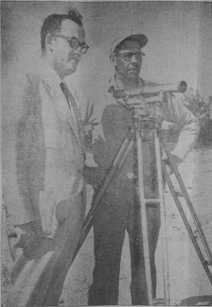
LOOKING OVER the site of the new Whittemore-Prescott Area School are John Halbert, superintendent of schools, left, and Clifford Morgan, superintendent of construction for Vollmer Construction Company.—Tawas Herald Photo.
