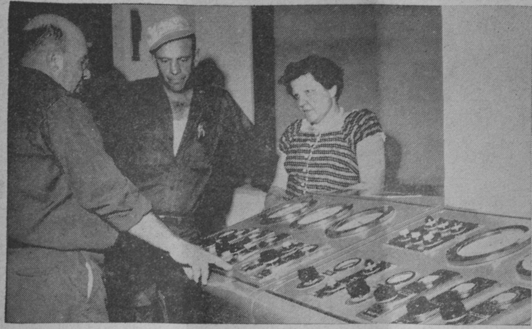
RESIDENTS OF THE TAWASES got a first-hand look of the new East Tawas filtration plant at an open house observation last Saturday. In this picture, Harry Cater shows two visitors some of the equipment at the plant.—Tawas Herald Photo.
