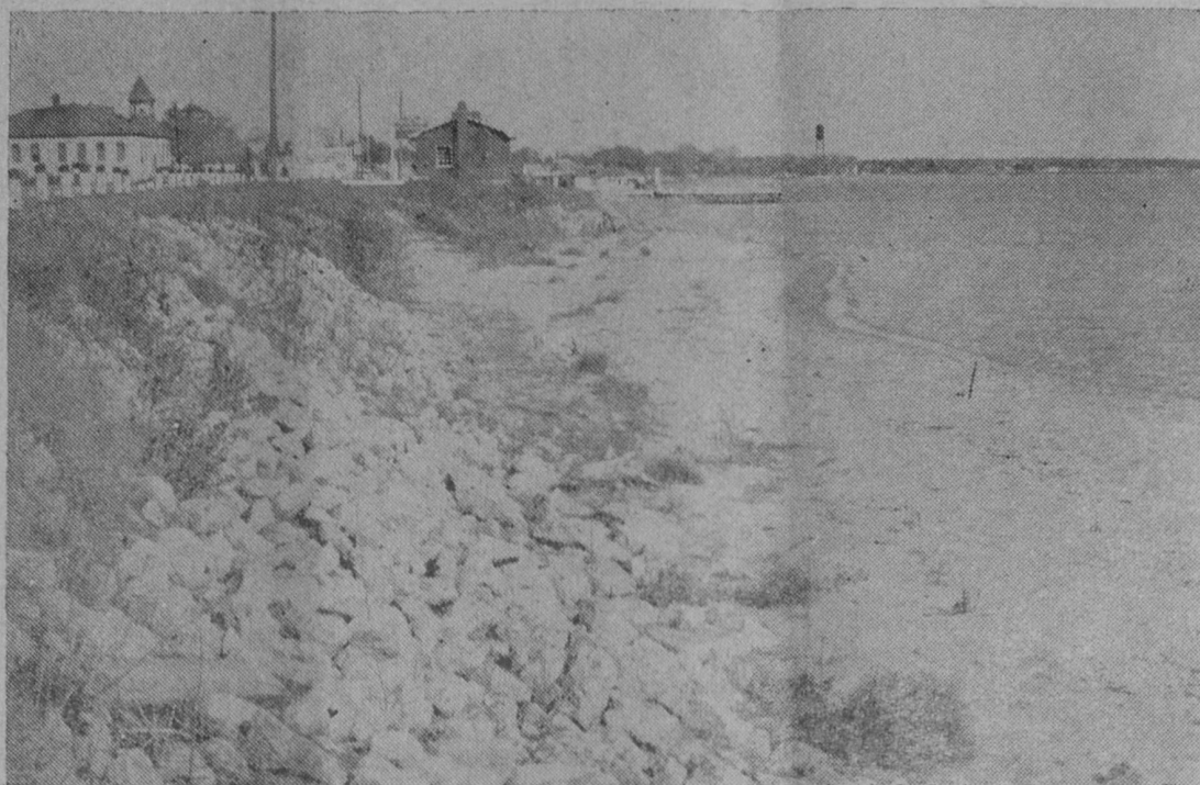
DO YOU REMEMBER when the picture at left was snapped? It was taken in the fall of 1952 when waters of Tawas Bay were washing away the shoreline, endangering US-23 at the intersection of M-55 in Tawas City. The City of Tawas City, with Martin Kasischke as superintendent of public works, installed a temporary break-wall to protect the shore from erosion in that area. The picture above shows this same area today. Since 1952, the water level of Lake Huron has dropped nearly four feet, leaving exposed rocks and long expanses of beach. Although local residents will tell you that the lake is at its lowest level in history, lake survey reports of army corps of engineers indicates that the lowest level was in 1934, when it was about a foot lower. However, this old record has probably been broken because the figures used here were in the September report. Highest recorded level was in 1876 when the water reached an elevation of 583.42 feet above the mean tide of New York, or .42 of an inch above the 1952 level.—Tawas Herald Photos.
