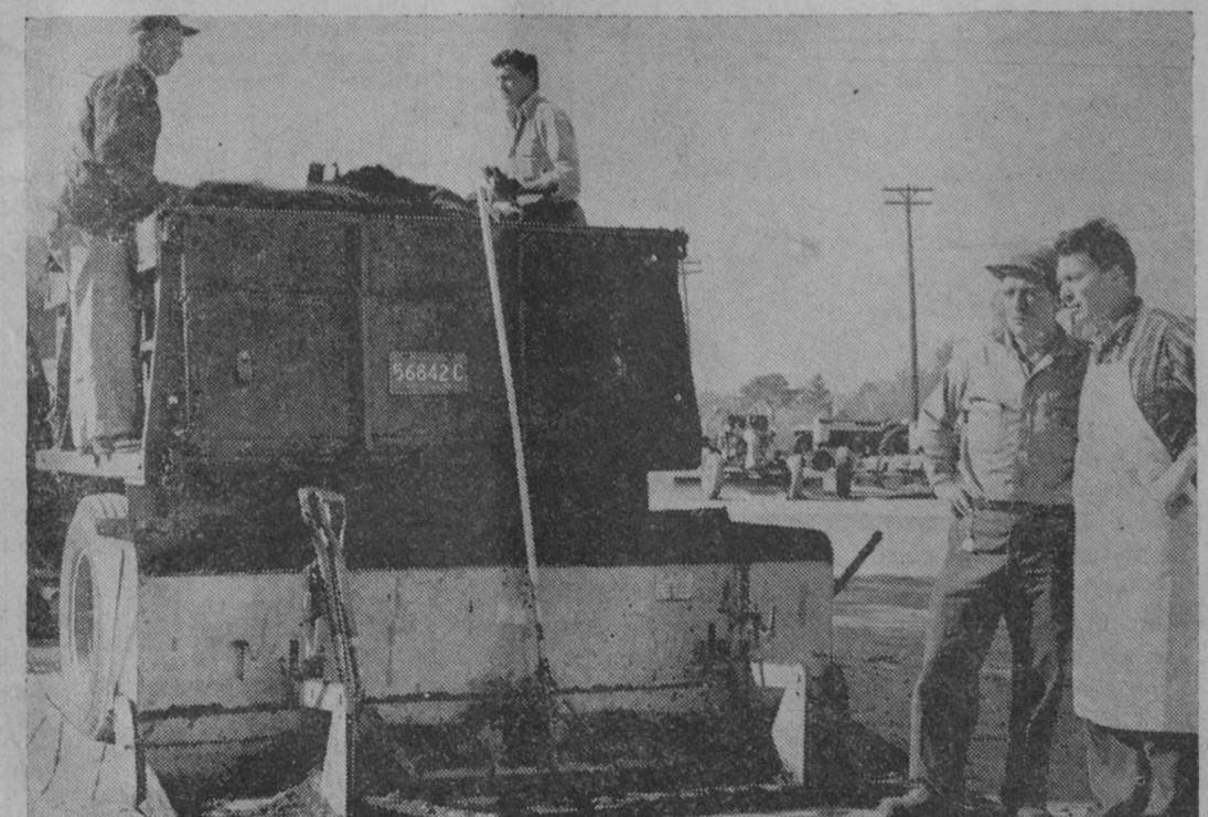
BRUGGER'S MARKET in Tawas City completed its new 35-car parking lot Monday. In the above picture, John N. Brugger is shown with Howard Hilderbrand while the lot was being black-topped. Hilderbrand of Oscoda was contractor for the work.—Tawas Herald Photo.
