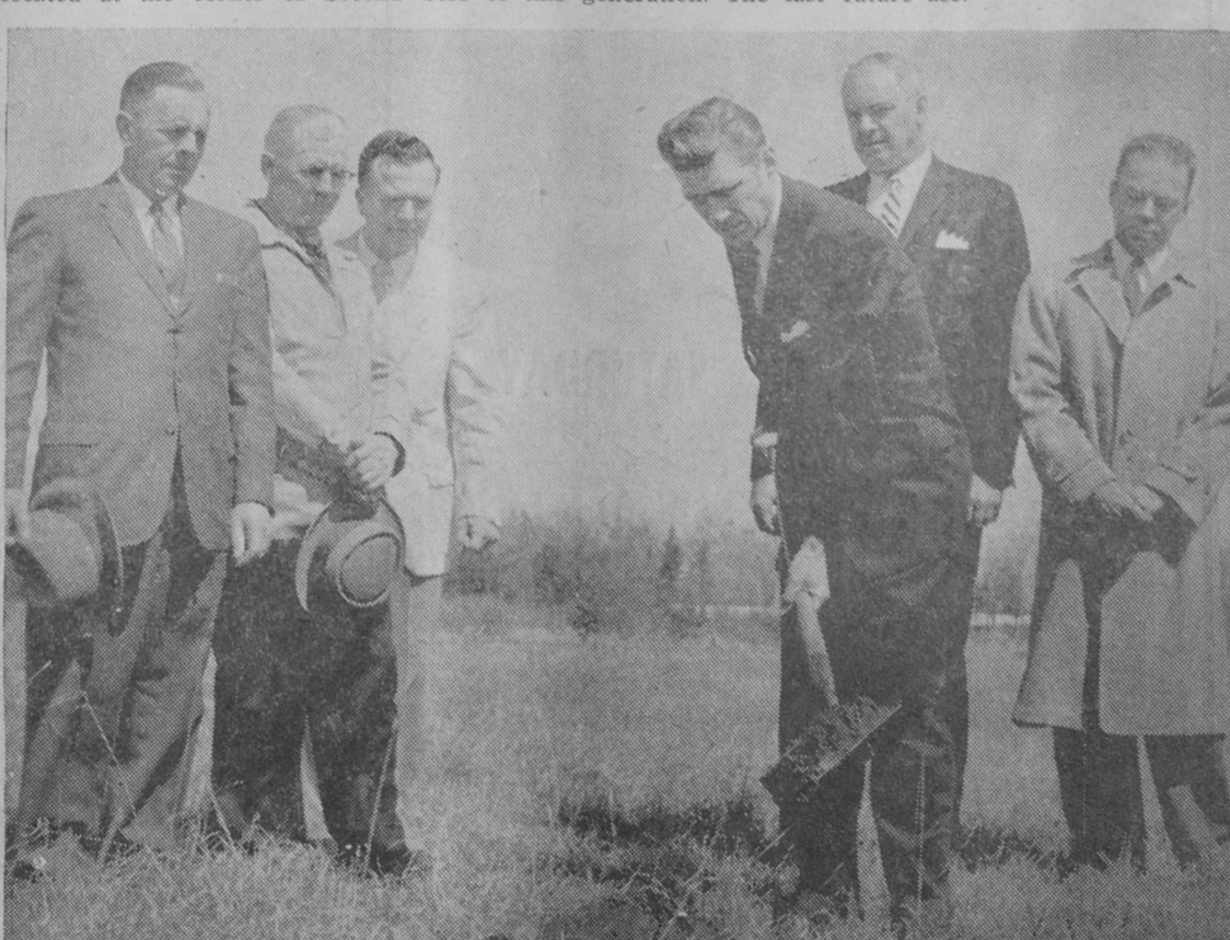
GROUND-BREAKING CEREMONIES for Emanuel Lutheran Church's new school were held last Sunday morning. In the above picture, the Rev. Leonard Newman turns over the first spadeful of sod. Watching, from left to right, are: William Look Sr., chairman of the building committee; John St. James, Arnold Hosbach, Joseph Fox and Frank Ahonen.—Tawas Herald Photo.
