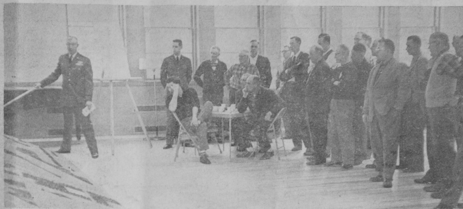
WITH THE AID of a scale model of Wurtsmith Air Force Base, Lt. Col. C. Hunter Smith, SAC liaison officer, left, points out locations of new facilities now under construction. Standing second from left is 1-Lt. David Morton, installation engineer, who outlined expansion plans which will take place during the next two years. At right are county supervisors and businessmen.—Herald Photos.
