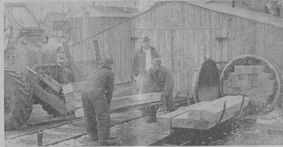
A CYLINDRICAL RETORT is being loaded in preparation for treating guardrail posts. Richard Sykes, inspector for the state highway department, stands at the rear as James Rapp and Irwin Shover load posts on a narrow gauge rail car. Tracks lead into the retort and one load can be seen at the entrance. About 15,000 guardrail posts are treated annually.—Tawas Herald Photo.
