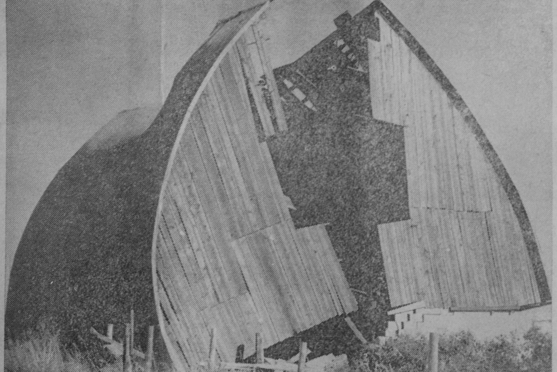
WEATHER CONDITIONS last week Wednesday were perfect for tornadoes in Northern Michigan, according to United States Weather Bureau. A cold front collided with a warm front and the result was a massive storm disturbance. This barn on M-55, seven miles west of Tawas City, owned by Hubert Klenow, was ripped apart by a heavy wind, but it is believed that the storm was not a "twister." Heading in a northeast direction, it destroyed a number of apple trees at the Charles Simons home. Accompanied by a driving rain, the blow lasted but a few minutes.—Herald Photo.
