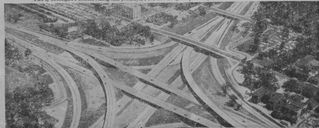
Two of Michigan's smooth-riding new freeways, Ford and Lodge Expressways, shown at Interchange in Detroit
