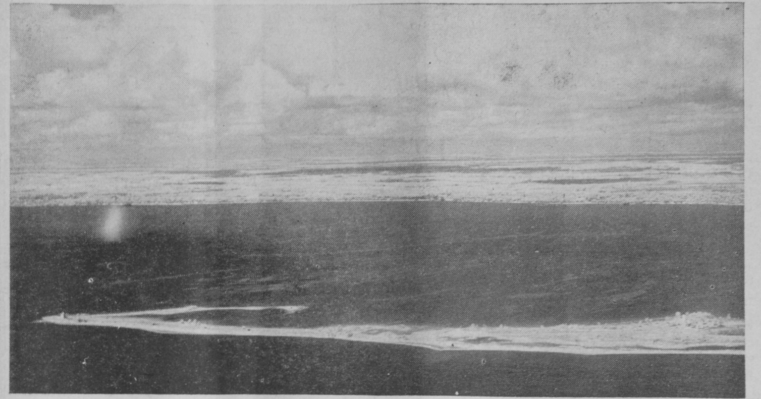
THE NARROW strip of land extending out into the black area in the above picture is the tip of Tawas Point, with Tawas Bay and the Tawas in the background and Lake Huron in the foreground. This aerial view takes in that part of the point which is now being considered for a public recreation area. The Tawas Point Lighthouse is near the right edge of the picture. Infrared film was used in the camera to "cut" the haze. This is the reason for the white foliage on Tawas Point and the background.—Tawas Herald Photo.
