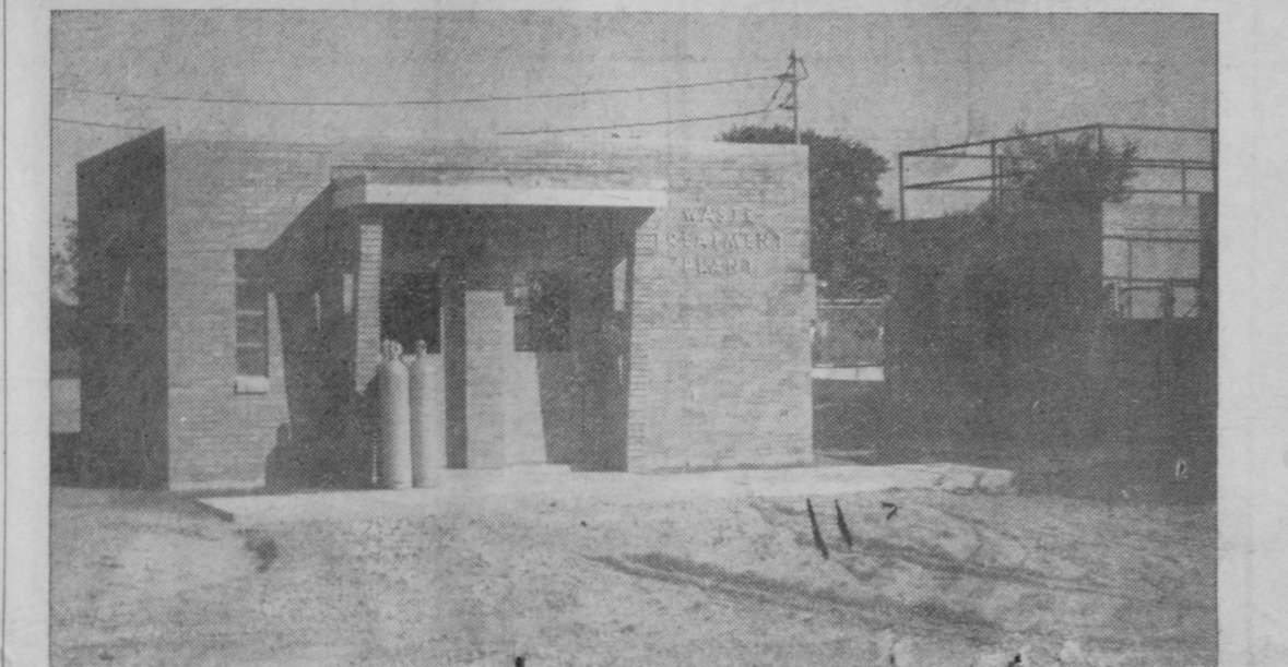
NEW BUILDING housing the laboratory and chlorination equipment at the Tawas City disposal plant is shown above. Included in a $112,609.40 addition to the disposal plant facilities, the laboratory has the latest equipment for protecting the health of area residents. Contractor for the project was B. H. Sargent Construction
