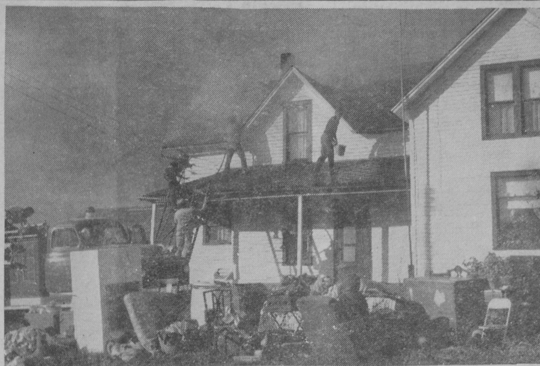
BURNING FARM HOME —Household articles owned by Mr. and Mrs. Howard Scholtz were stacked up in front of their home west of Whittemore last Thursday as firemen and volunteers battled to save the burning structure. Fire, smoke and water caused extensive damage to the building. Cause of the blaze was unknown but was believed to have started in the attic or roof. Workmen from the nearby Chamabi Ranch kept the flames under control until arrival of the Whittemore Fire Department. The Prescott Fire Department was called later. This was the second time in less than two years that the Scholtz family has been routed from their home by fire. All of their household belongings and clothing were lost January 28, 1959, when their home burned on Meadow Road, west of Tawas City.—Tawas Herald Photo.
