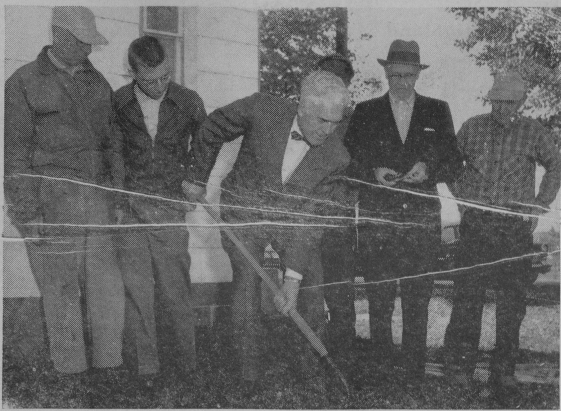
GROUND WAS broken last week for a new addition to the Seventh-day Adventist Church at the corner of Tawas and Adams Streets in East Tawas. Shown with the shovel is the Rev. Herbert Alexander, pastor. Watching from left to right are Kenneth Sherman, Earle Doughty, Edson Lewis (behind Mr. Alexander), Walter Mason and William White. The new 24 by 20 addition is to house extra classrooms and rest rooms. The front of the building will be modernized with a tinted glass window. Mason, who is conference builder, will be in charge of construction.—Tawas Herald Photo.
