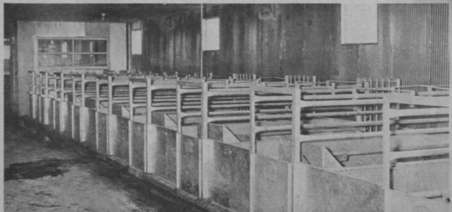
There are 20 farrowing stalls in the front half of the building, 10 on a side. The rear section of the building is occupied by 10 weaning stalls. A radiant heating system in the floor insures that the pigs are comfortable on the coldest days.
